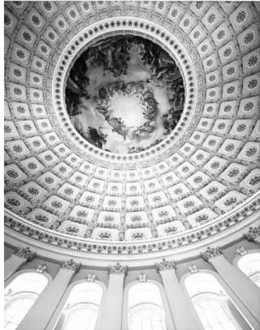
(The Inner Dome and Canopy over the Rotunda)
